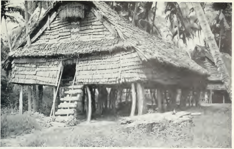
A. Dwelling house in Kankanamun village
